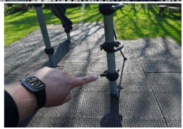
**Finding:** The rubber covering has been damaged exposing **Action**: Repair or replace rusty steel
