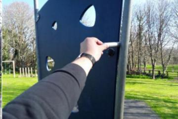
Finding: There is/are finger entrapment/s in the frame and Action: Monitor - No remedial work recommended the item fails to meet the requirements of BS EN 1176 Part 1 4.2.7.6 Entrapment of fingers
