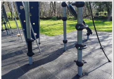
**Finding:** The multiple has missing component(s) on the structure
