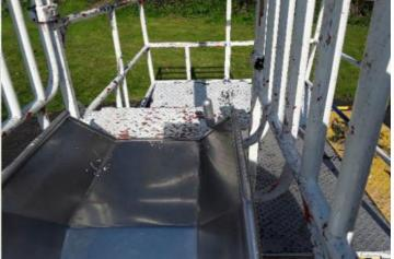
Finding: There is/are finger entrapment/s in the frame and Action: Monitor - No remedial work recommended the item fails to meet the requirements of BS EN 1176 Part 1
