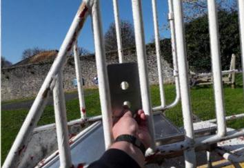
Finding: The item fails to meet the requirements of BS EN Action: Monitor - No remedial work recommended 1176 Part 1 4.2.7.2 for head and neck entrapment in the
