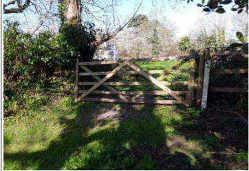
**Finding:** The gate post has rotted and sheared and is unstable, the additional support posts installed are inadequate to support the structure.
