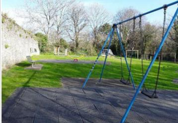
Finding: The safety surfaces around the site have been damaged/are wearing
