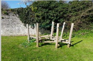
**Finding:** The connecting links are in excess of 8.6mm and less than 12mm and fail the requirements of BS EN 1176
