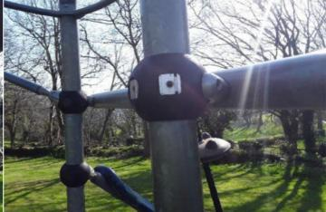
**Finding:** There is/are finger entrapment/s in the frame due to missing fixings and inserts and the item fails to meet the requirements of BS EN 1176 Part 1 4.2.7.6 Entrapment of fingers
