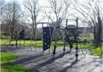
**Finding:** There is/are finger entrapment/s in the frame due to missing inserts or fixings and the item fails to meet the requirements of BS EN 1176 Part 1 4.2.7.6 Entrapment of fingers
