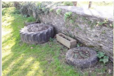
**Finding:** The tyre planter may encourage access onto the top of the wall where there are falls of up to 1.8m to the surface outside of the play area.
