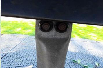
Finding: The fixings have corroded excessively
