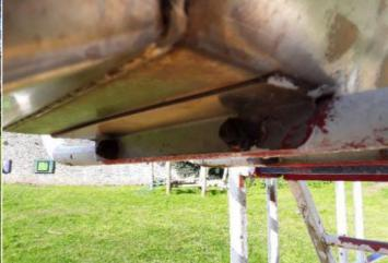
Finding: The fixings have corroded excessively
