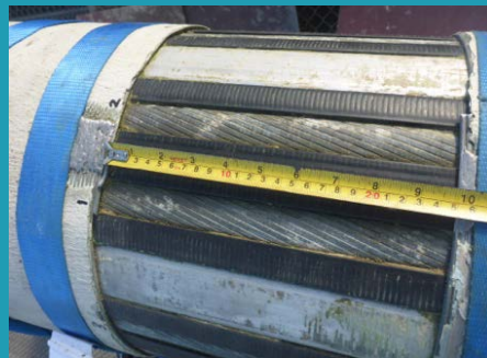
Typical unwrapped section of main cable showing wire ropes and cable fillers
